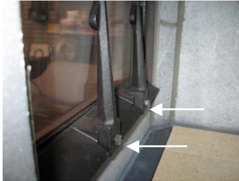
3. Using a 1/2" wrench, or socket and ratchet, carefully loosen the bolt at the base of each andiron and remove them.
