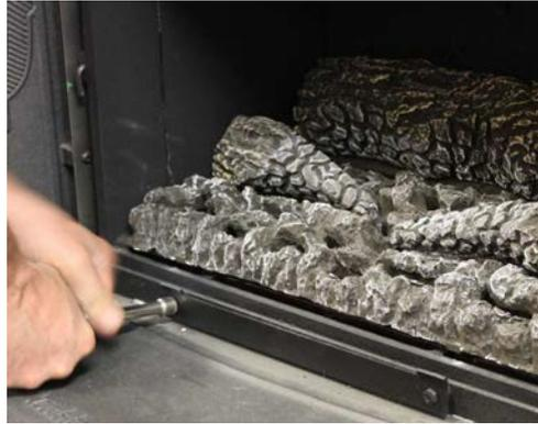
4. Remove the bolt that holds the burner in place. It is at the bottom center of the firebox and will be visible once the glass retainer is removed.
