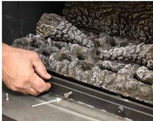
5. Very carefully remove the log set. It is very fragile and should be supported with two hands under the base. If the base of the log set is damaged the log set should be replaced.
